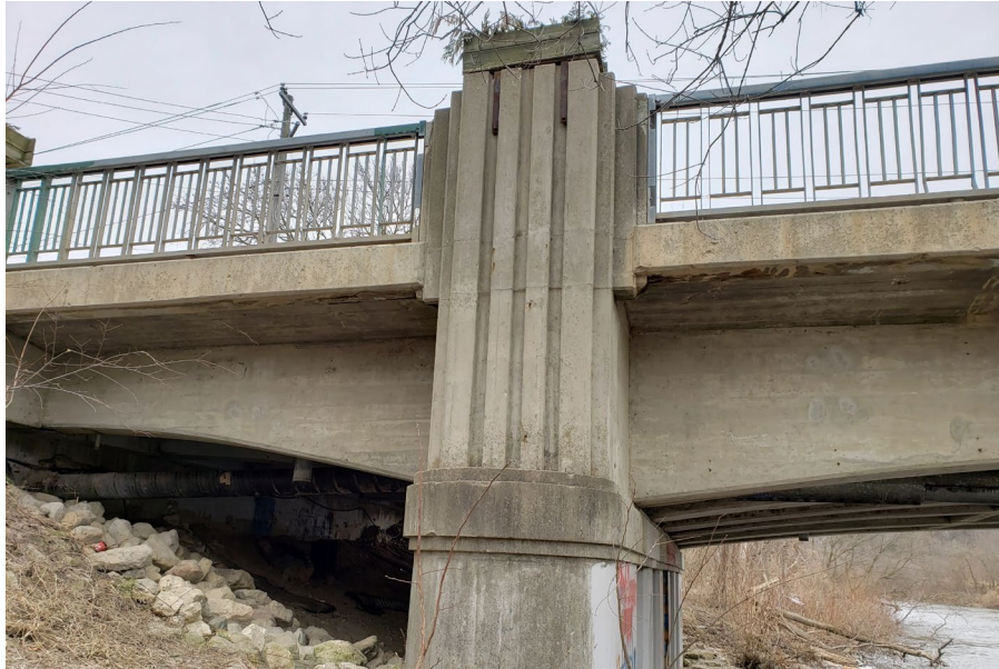
Image 22: Exterior view of stanchion/pillar with embossed detailing (TMHC 2021)
