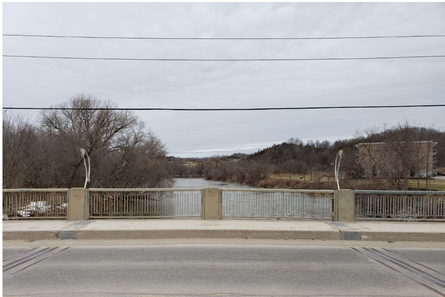
Image 13: North side (interior) of Durham Street Bridge (TMHC 2021)
