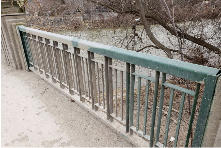
Image 30: Railing detail (TMHC 2021)
