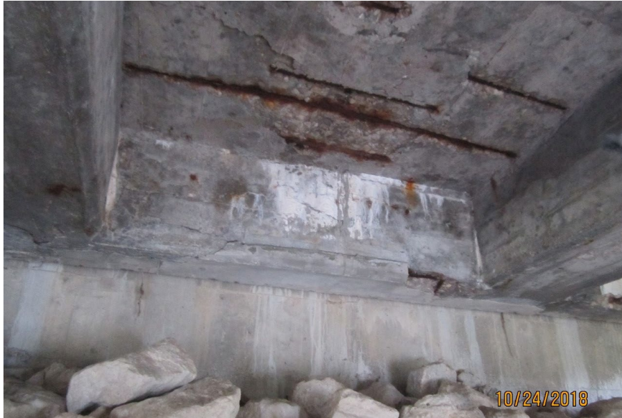
Image 45: North diaphragm and soffit (image provided by BM Ross 2018)
