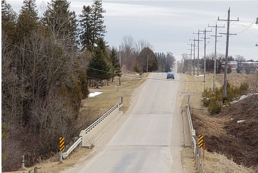
Image 44: Nearest bridge upriver - South Durham Road/Concession 2 (TMHC 2021)
