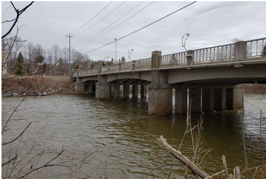
Image 17: North piers and stanchions (TMHC 2021)
