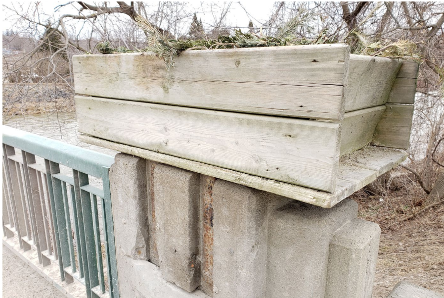
Image 25: Planters box in former light standard location on top of stanchion (TMHC 2021)
