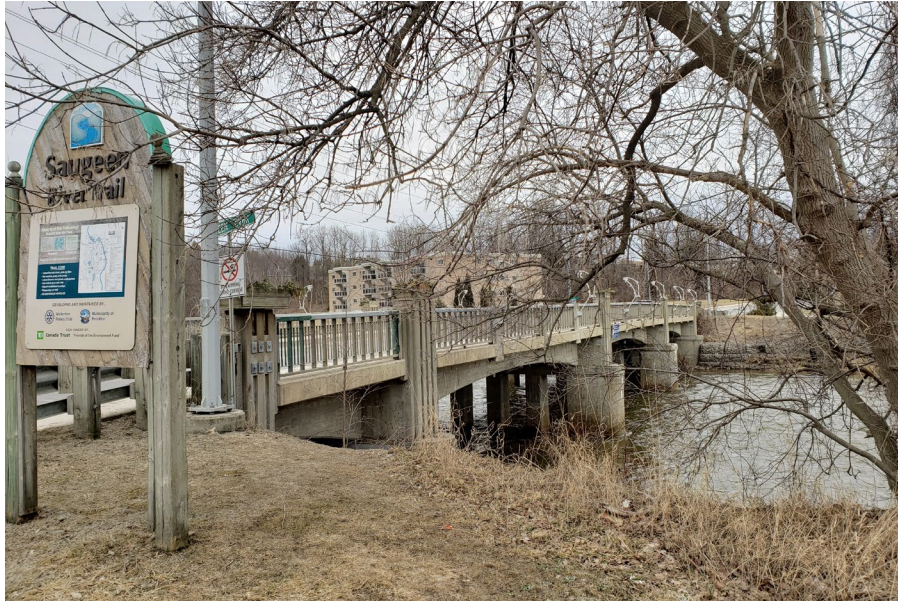
Image I4: South side (exterior) of Durham Street Bridge with trail sign (TMHC 2021)
