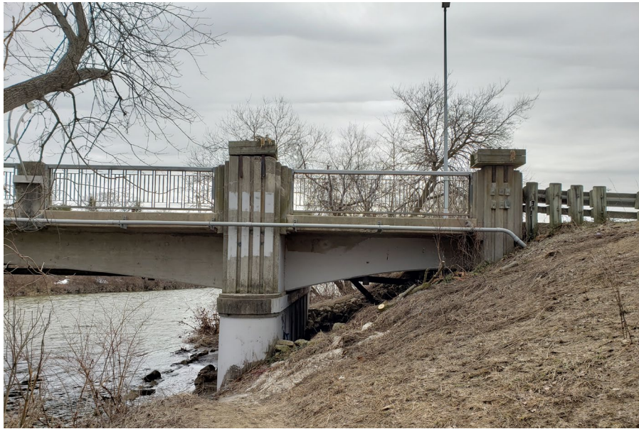
Image I9: Short cantilevered west approach span (TMHC 2021)
