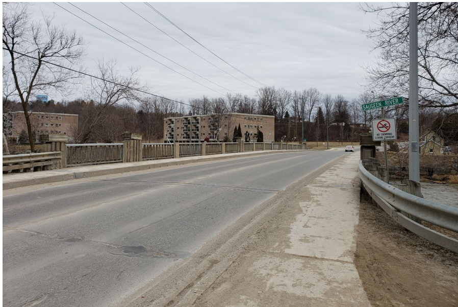
Image 9: West side of Durham Street Bridge (TMHC 2021)
