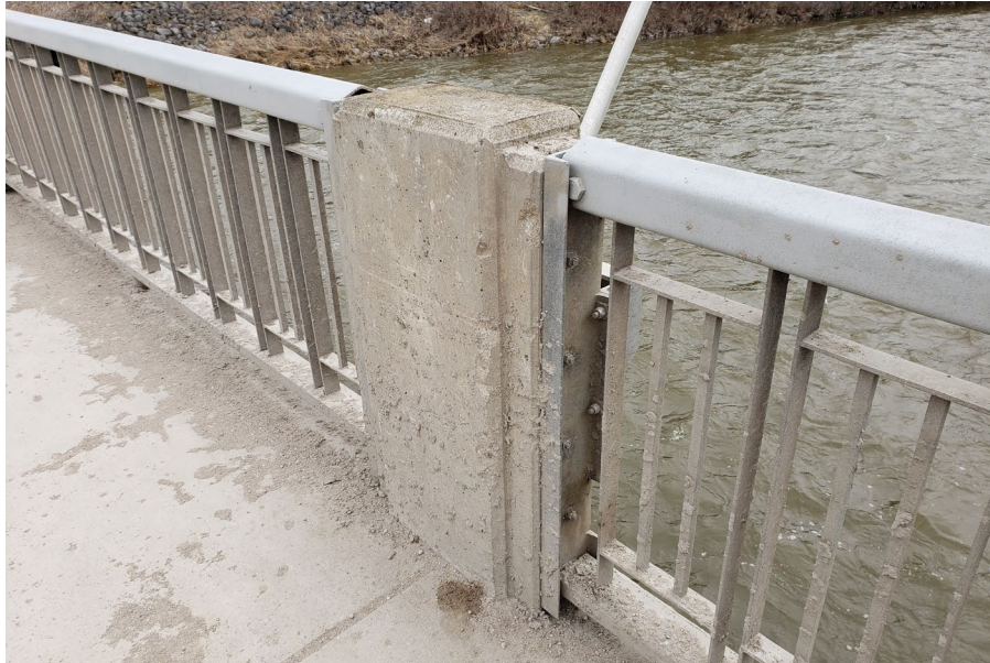
Image 26: Concrete railing post (TMHC 2021)
