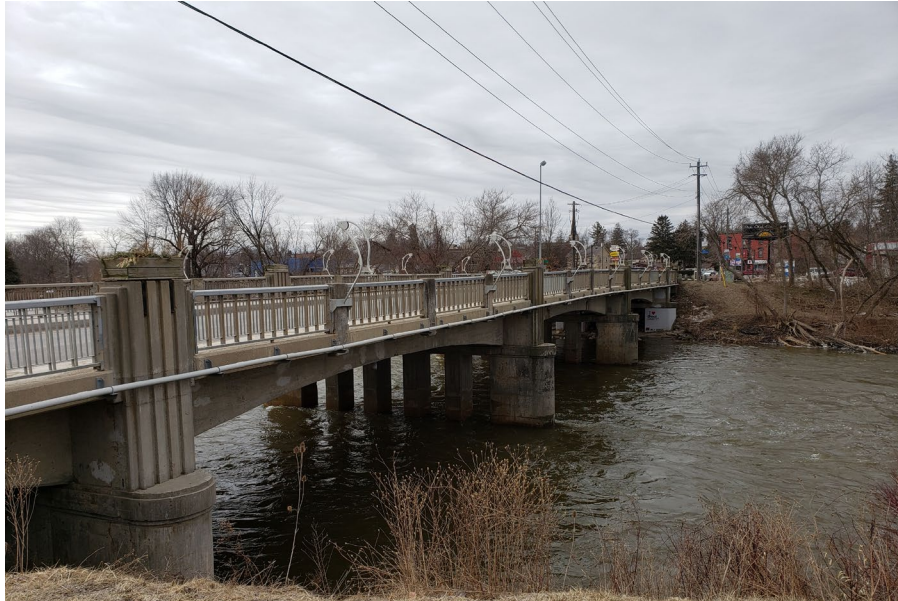
Image 12: North side (exterior) of Durham Street Bridge (TMHC 2021)
