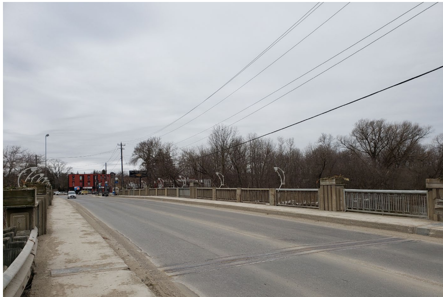
Image 11: East side of Durham Street Bridge (TMHC 2021)
