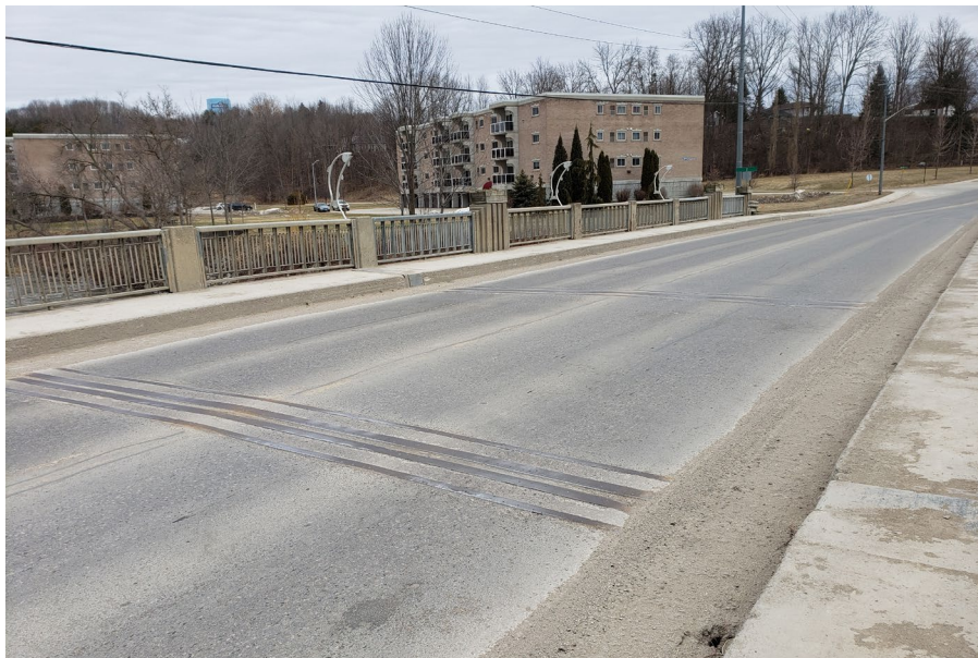
Image 21: Bridge deck at drop-in center span (TMHC 2021)
