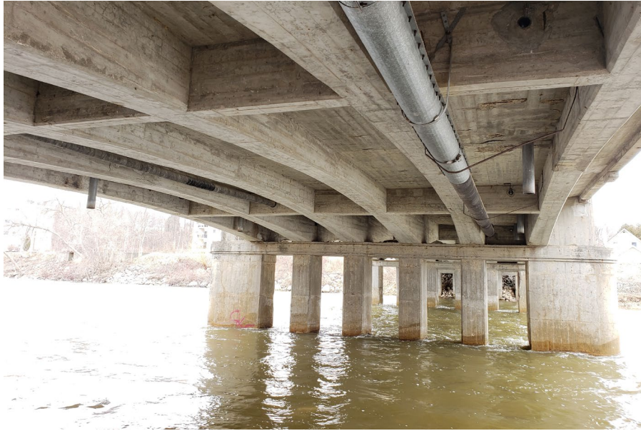
Image 16: Bridge soffit (TMHC 2021)
