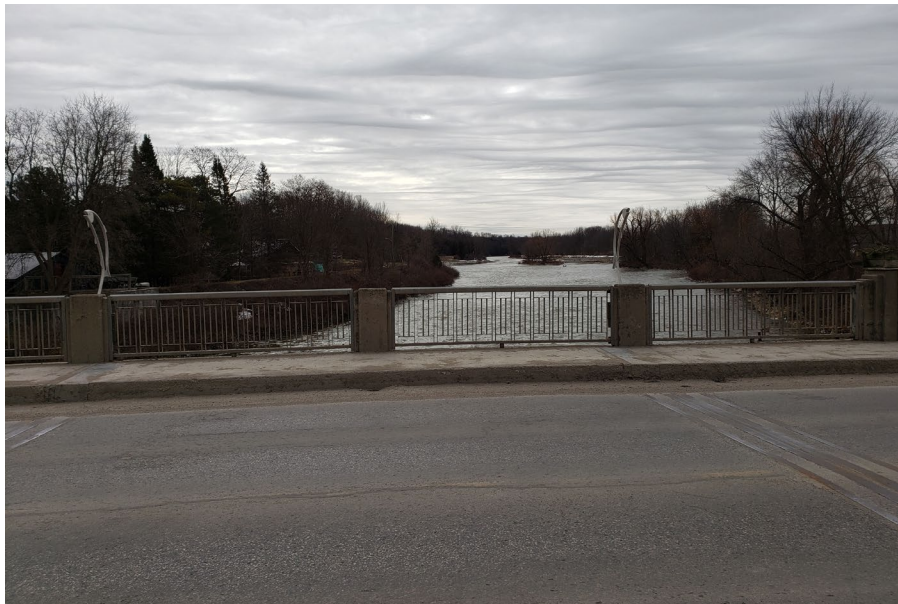
Image I5: South side (interior) of Durham Street Bridge (TMHC 2021)
