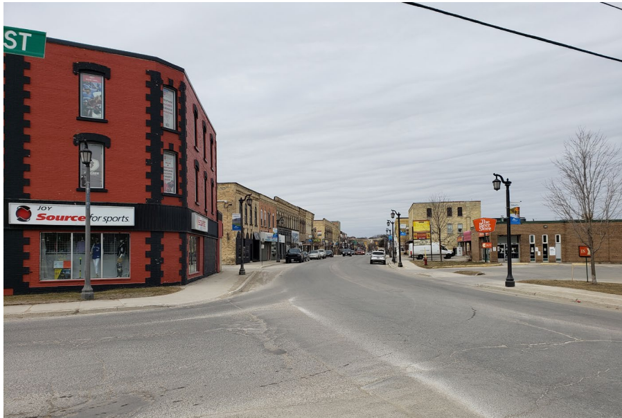
Image 40: Durham Street into Historic Walkerton - west of Durham Street Bridge (TMHC 2021)
