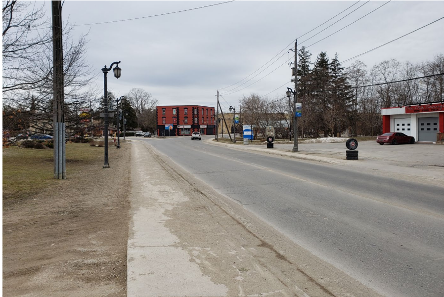
Image 8: Westward approach to Durham Street Bridge (TMHC 2021)
