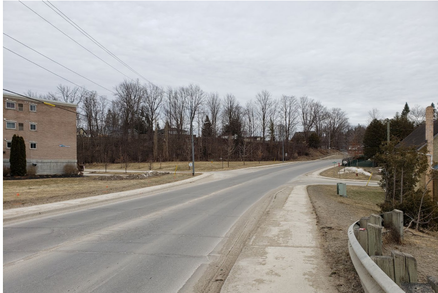
Image 10: Eastward approach to Durham Street Bridge (TMHC 2021)
