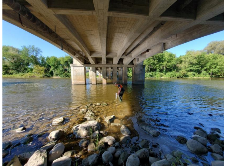
East side of bridge, view from bank facing west ↑
