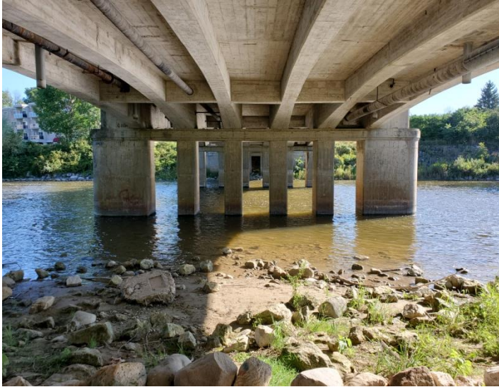
West side of bridge, view from bank facing east ↑
