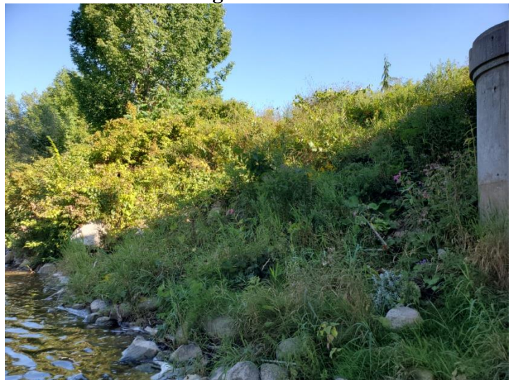
Vegetation on northeast bank of bridge ↑
