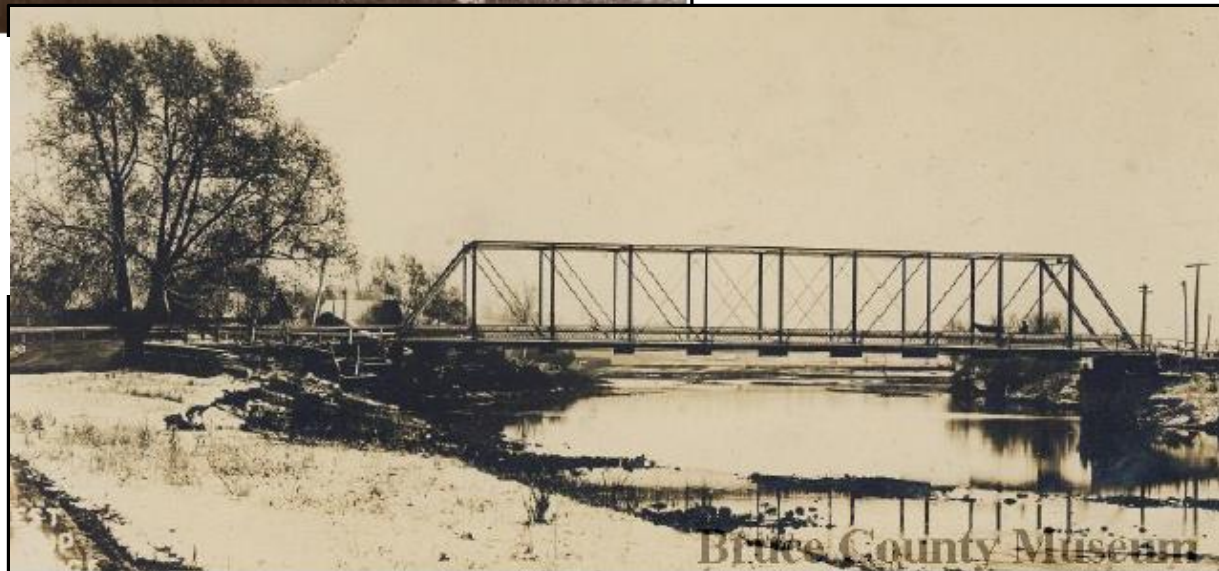
Image 5: Previous truss bridge in 1908 (Bruce County Museum & Cultural Centre)
