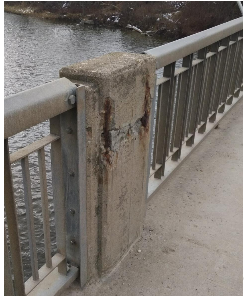
Concrete deterioration
