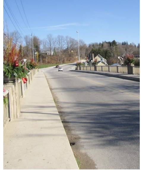
ACCESS OVER RIVER DURING CONSTRUCTION
