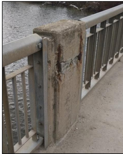
CONCRETE DETERIORATION
